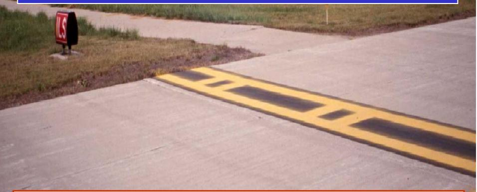
At some airports it may be necessary to hold an aircraft on a taxiway at a location other than at the runway entrance if the ILS is in use. Holding the taxiing aircraft at the ILS hold point will preclude ILS signal interference with an aircraft on ILS final approach.
