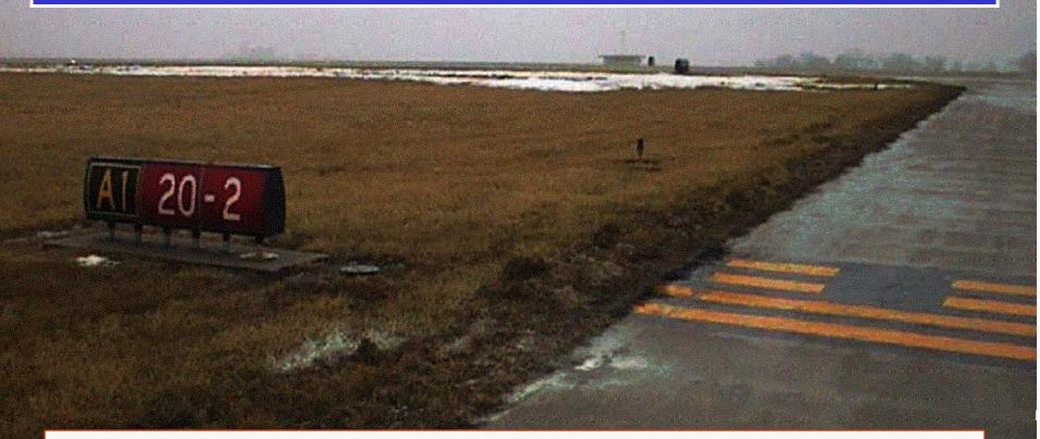
Note: This sign is located at the holding positions on taxiways that intersect a runway or on runways that intersect other runways. The runway numbers are arranged to correspond to the respective runway threshold. For example: "20-2" indicates that the threshold for Runway 20 is to the left and the threshold for Runway 2 is to the right.
